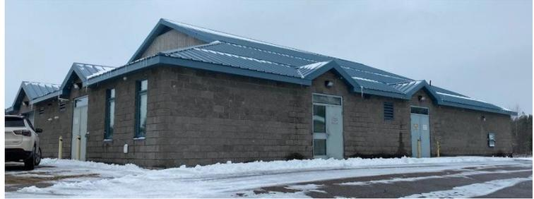
provides full conventional treatment to raw water drawn from the South River. The water treatment facility consists of two (2) Conventional Napier Reid package plants. An in ground clear well reservoir located under the facility has the approximate capacity of 1,536 m<sup>3</sup> of useable storage. High lift pumps at the treatment facility run continually to maintain water pressure in the water distribution system piping.
